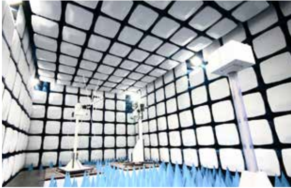
전무반사실 Fully Anechoic Chamber
